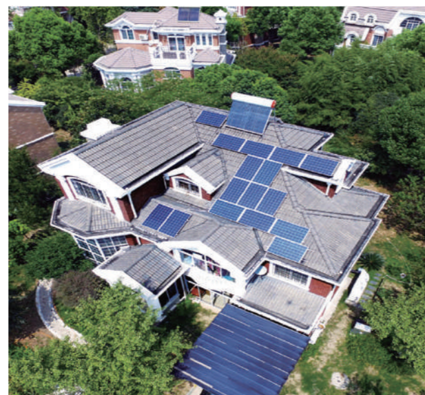
Residential Project in Philippines 3kW
