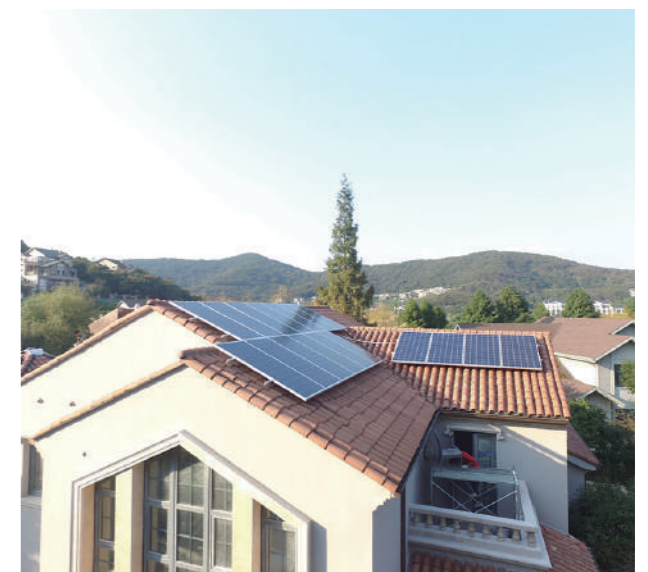
Residential Project in Argentina 5kW
