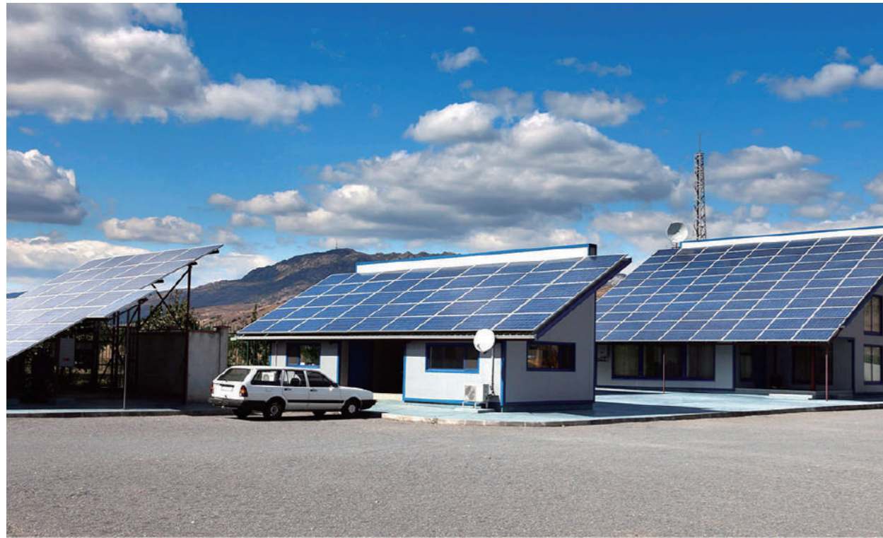
Residential Project in Indonesia 6kW
