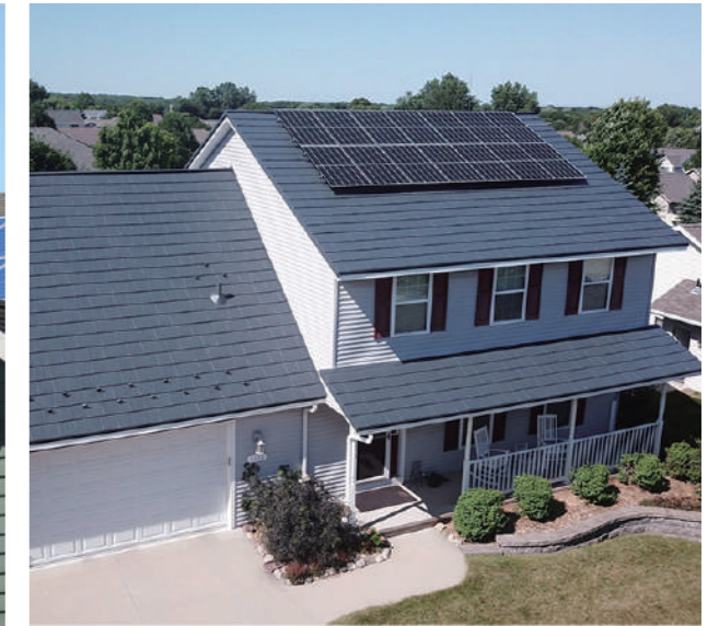
Residential Project in Philippines 3kW
