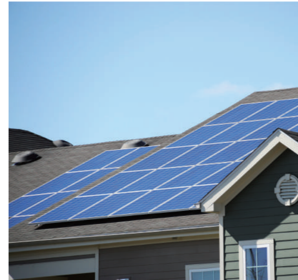
Residential Project in Indonesia 6kW
